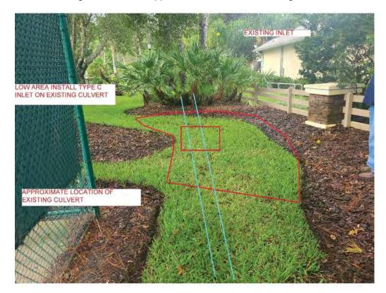
2. Photo showing existing inlet 205 located southwest of the tennis courts. Inlet is located within the mulched area and we recommend installing a steel mesh screen over the existing grate to deter mulch from entering and clogging up the drain and minimize future maintenance.
